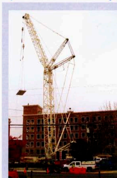
PRECAST ERECTION in Winchester
